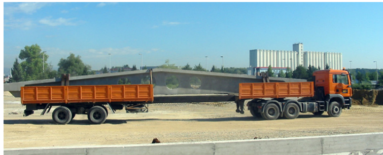
Figure 7. – Roof girder transportation
