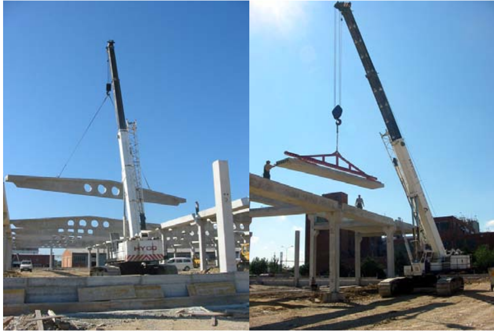
Figure 8 – Roof girder assembly; Figure 9 - Floor slab assembly
