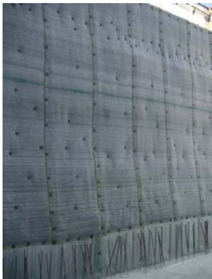
Placing into the formwork and a completed wall. Fig. 4 and 5.
