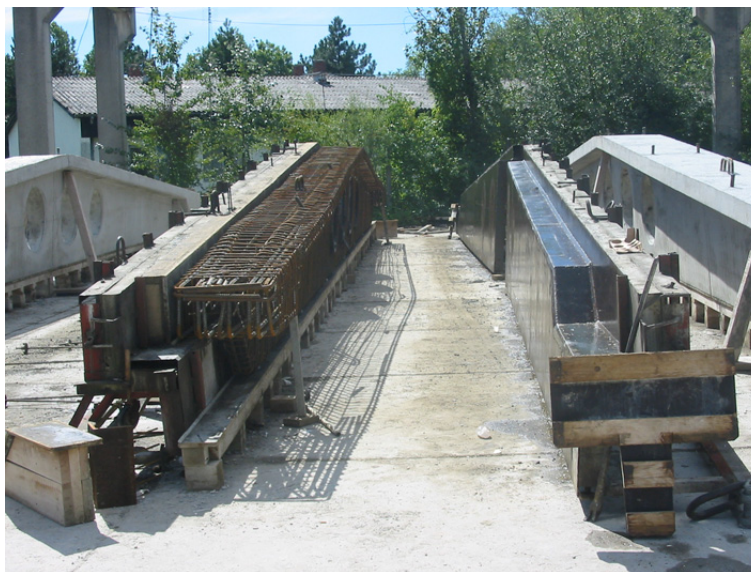
Figure 6 – Steel-plated mould - opened
