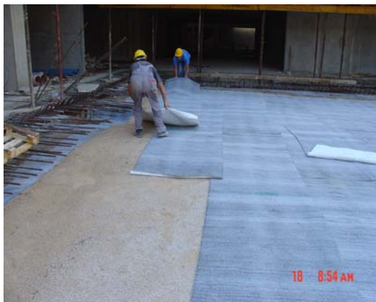
Fig. 3. Presentation of the placement on the foundation.
